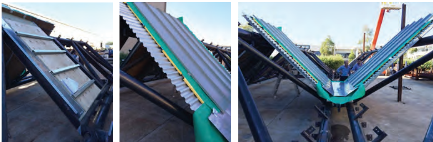
Figure 5 Structural steel fabricator's off site prototype mock up.
