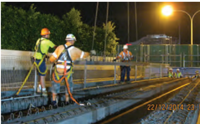
Figure 3 Workers on harnesses install the transfloor panels
