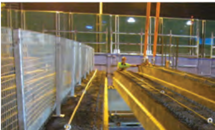
Figure 4 Precast planks installed from Peri scaffold system
