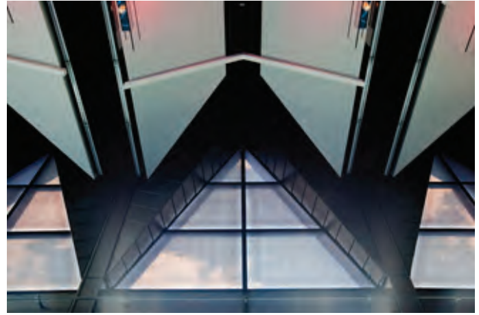
Figure 9 Triangular glazing with electro-chromatic operation
