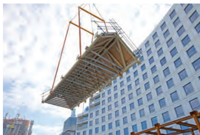
Figure 7 Prefabricated structural steel roof trusses being lifted into place.
