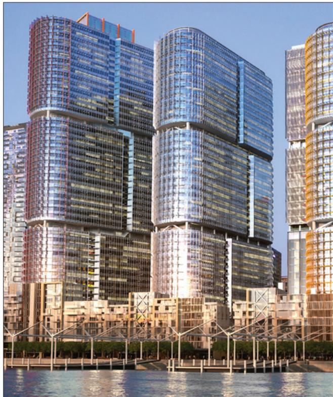
Figure 11. Each of the commercial towers has a three-lift rise format, and floor-to-floor levels are set at 3.8 m giving the 50-storey northern tower (left) an overall height of 210 m above ground
