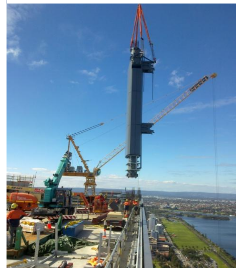
Figure 5 - Installation of pre-clad Capitol column
