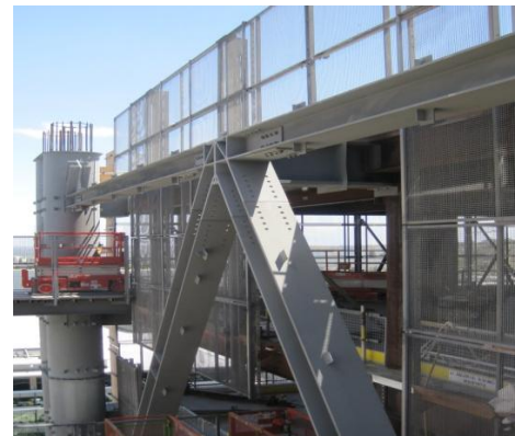
Figure 3 - K-Frame Steelwork Installation
