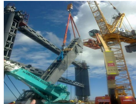
Figure 4 - Installation of Capitol Steel
