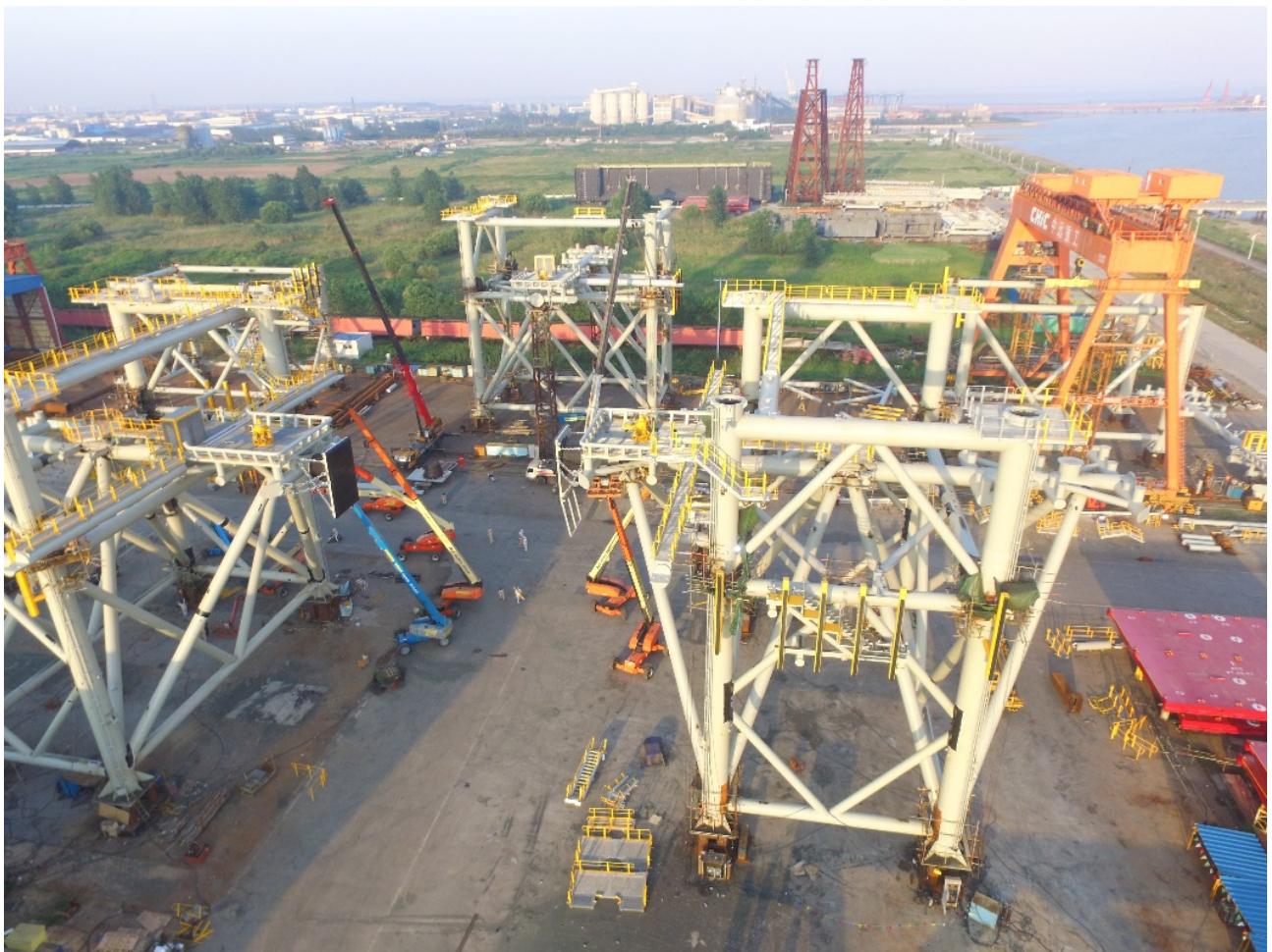
Picture – Fabrication of 30m-high jacket modules
