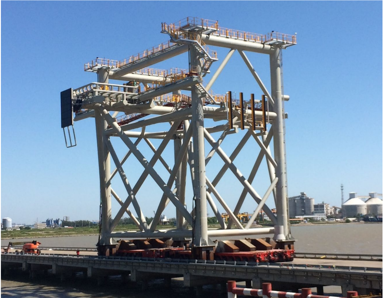
Picture – Transport of jacket structure at fabrication facility
