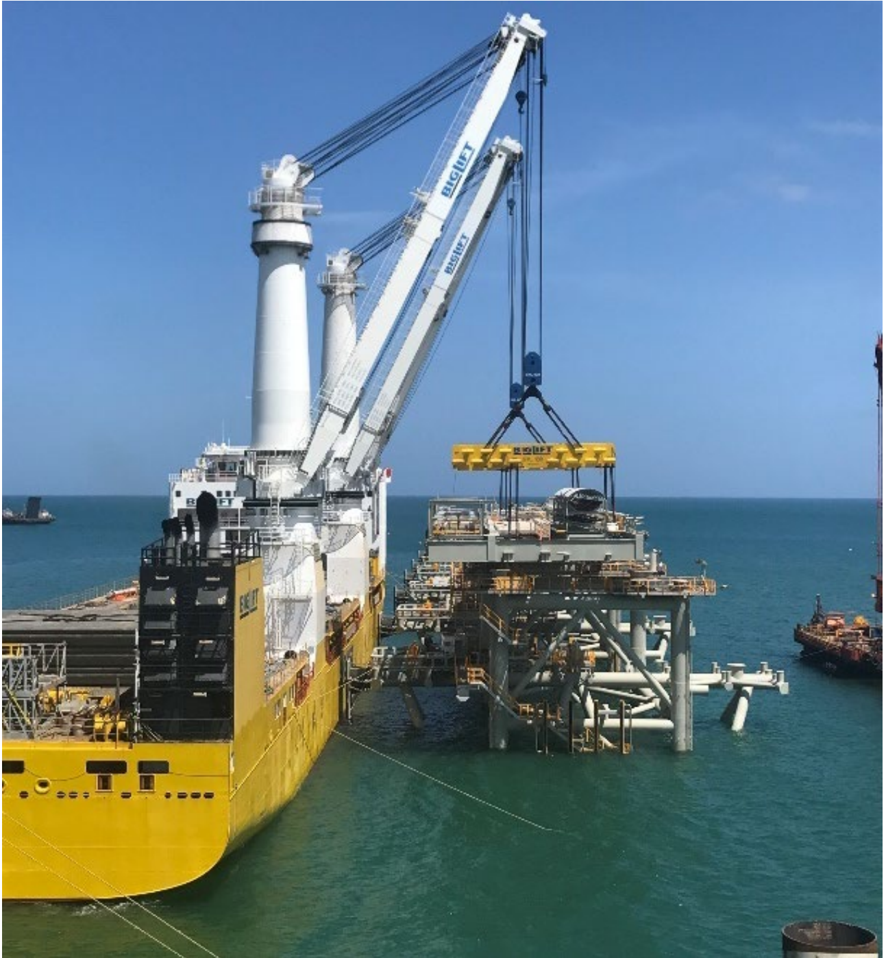
Picture – Heavy-lift ship placing modules
