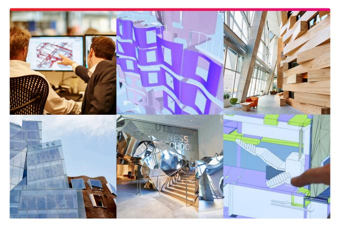
BIM was the vital tool that helped the construction teams to take the design from concept to reality. With the modelling technology, the construction teams could break complex designs into constructible parts, achieve extreme degrees of accuracy when putting them together, and better detect potential clashes.
