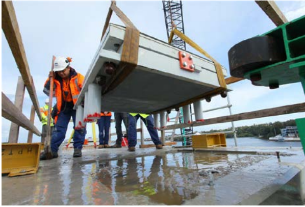
Bearings being lifted on top of pier
