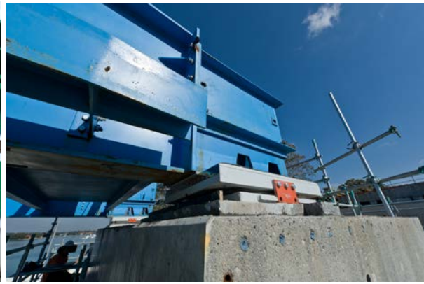
Bearings in temporary position during launching
