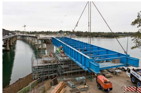
Launch nose dismantled by section as it passes over Pier 9
