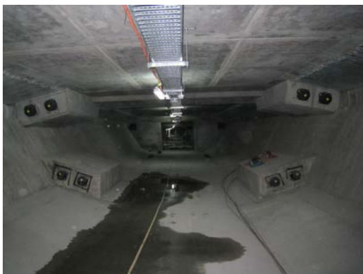
Stressing blisters inside box girder
