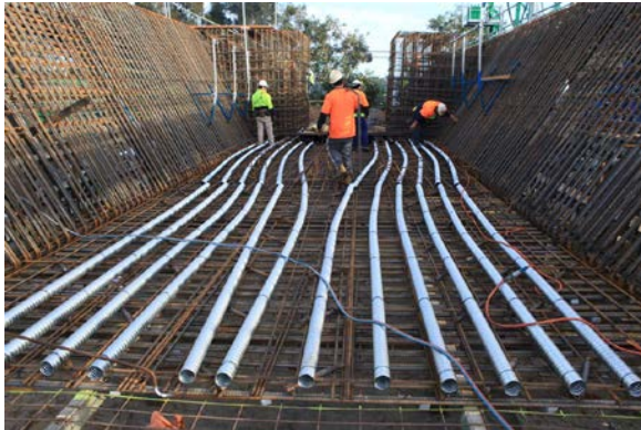
Rebar Jig installation of Bottom ducting
