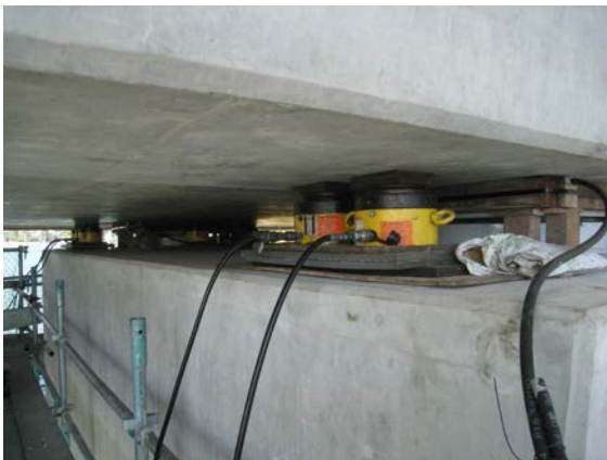
Relocation of pot bearings
