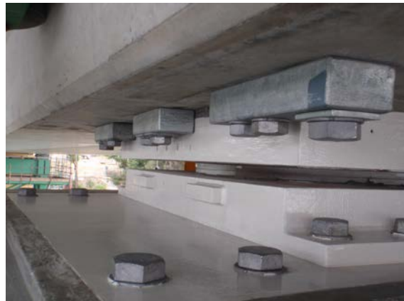
Bearings in permanent position with keeper plates installed
