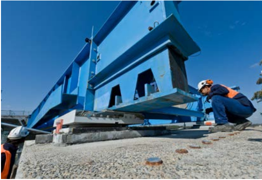
Launch nose jacking box on the bearings
