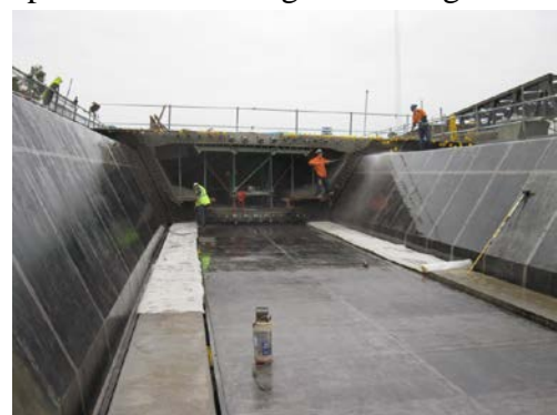
Casting bed preparation
