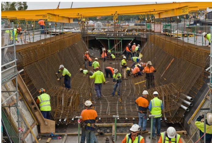
Rebar cage installation
