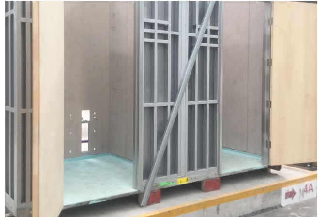
Image 18: Bathroom pods were used within the four accommodation buildings.
