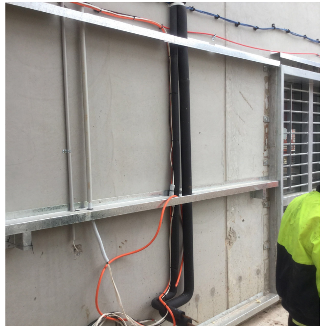
Image 19: Reticulated services were installed via a cavity between the precast wall and cladding.
