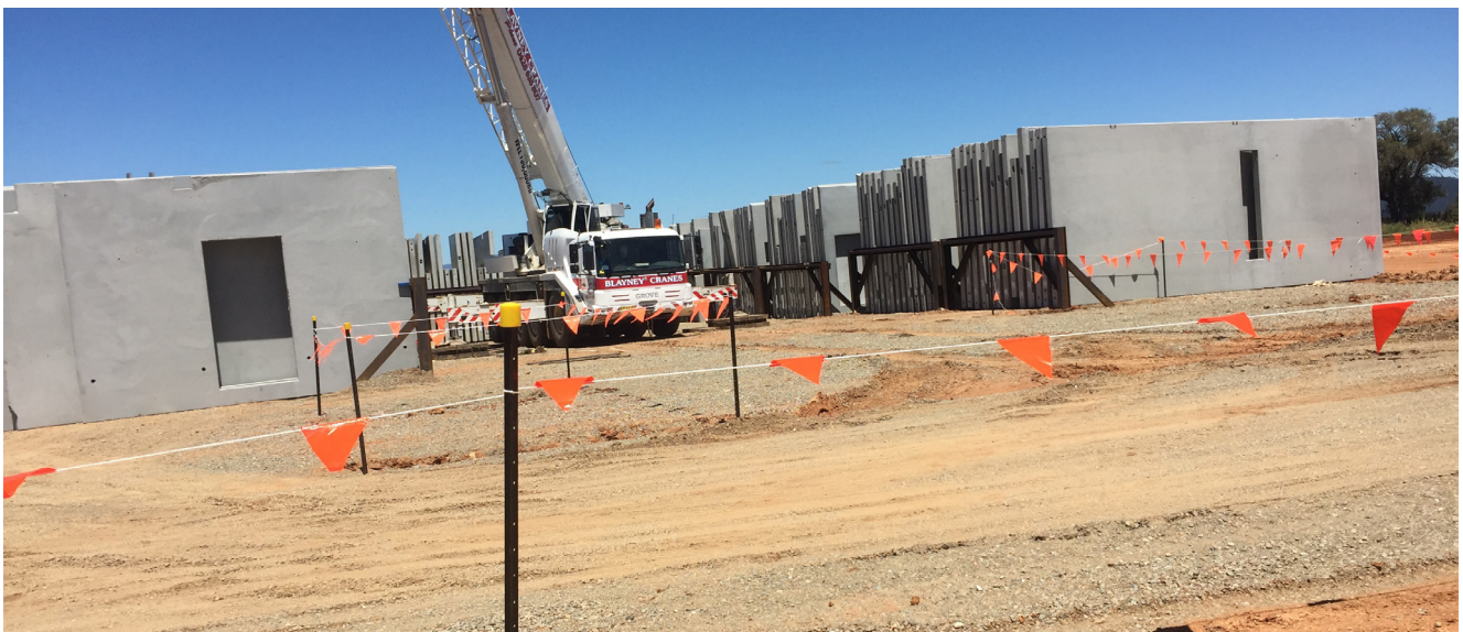
Image 20: Toaster racks were utilised on-site to stockpile precast walls to speed up construction.
