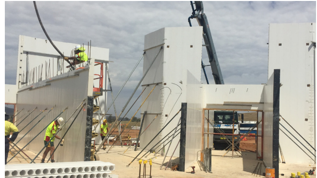
Image 10: Dincel was used for the central support building.
