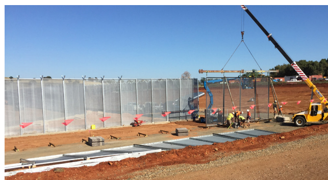
Image 15: Prefabricated security fencing was used for the 5.4km fenced perimeter.
