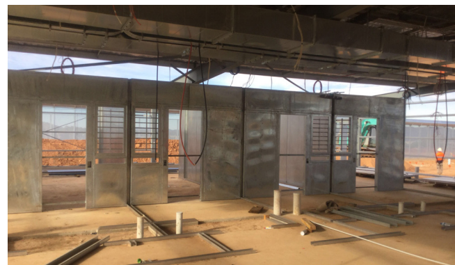
Image 13: Modsec was used for the segregation cells.
