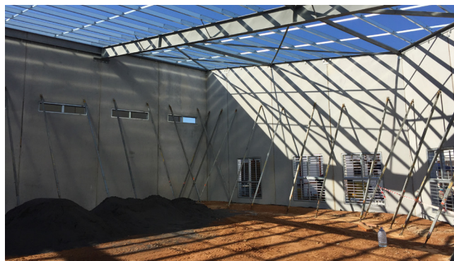
Image 14: Structural precast was used for the accommodation buildings.
