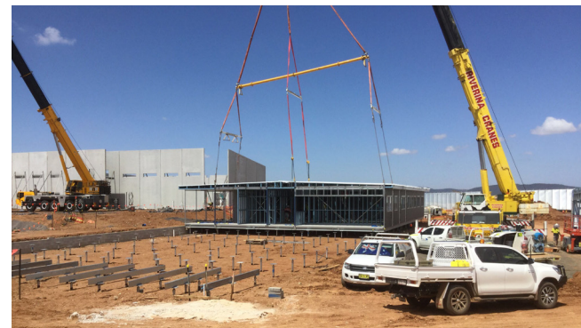
Image 12: Modular building systems were used for four entire buildings on-site.
