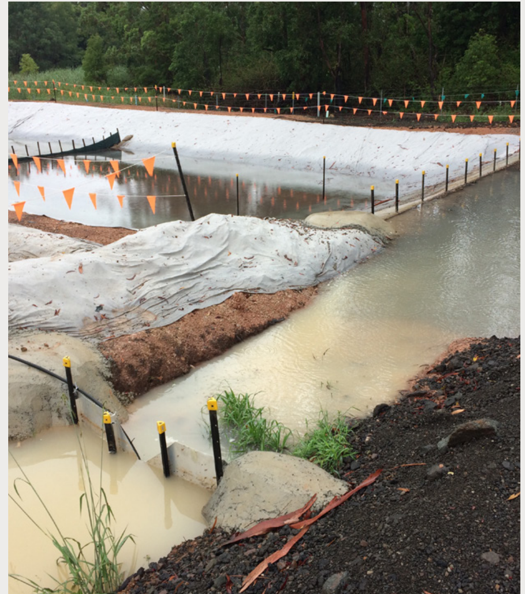
High efficiency self-dosing sedimentation basins were successfully trialled on the project.
