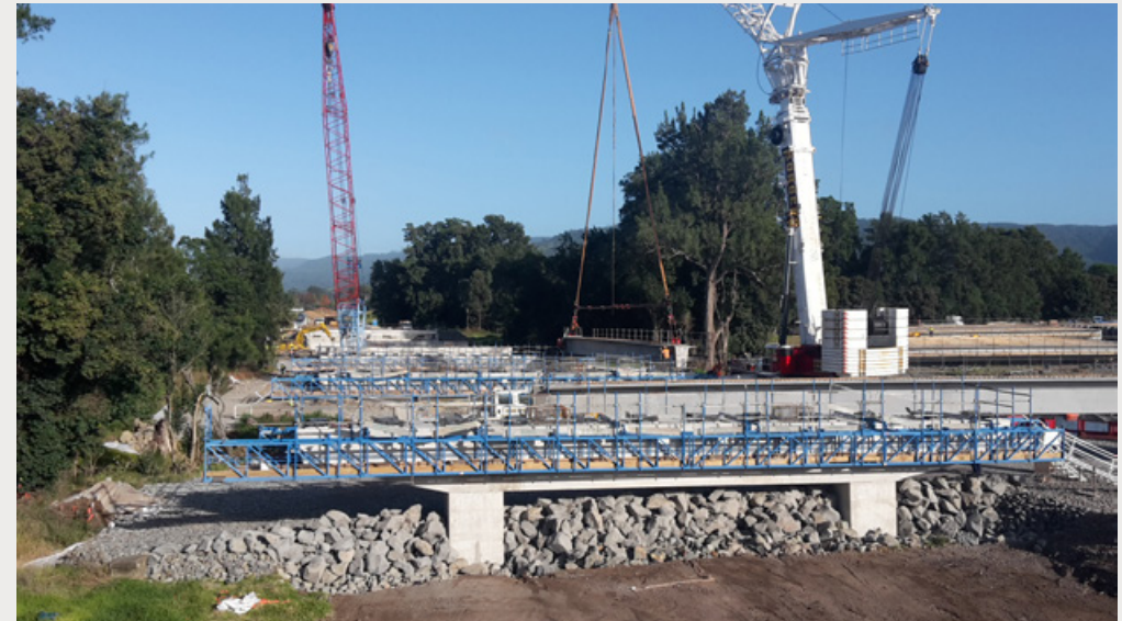
Super-T girder installation at Broughton Creek bridge three
