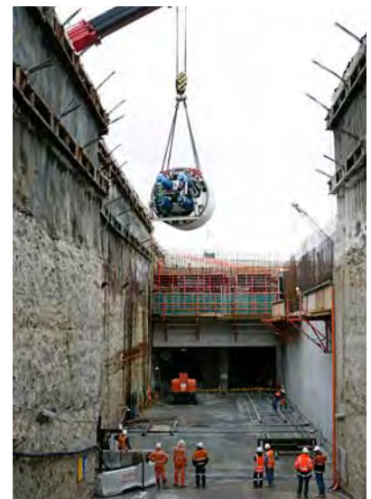
The first of the TBM components is lowered into the Box Cut.
