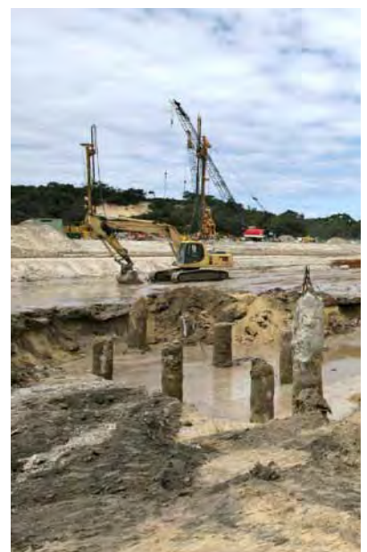
Pre-treatment Filters piling and excavation
