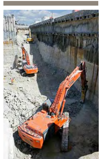
Excavating the Box Cut
