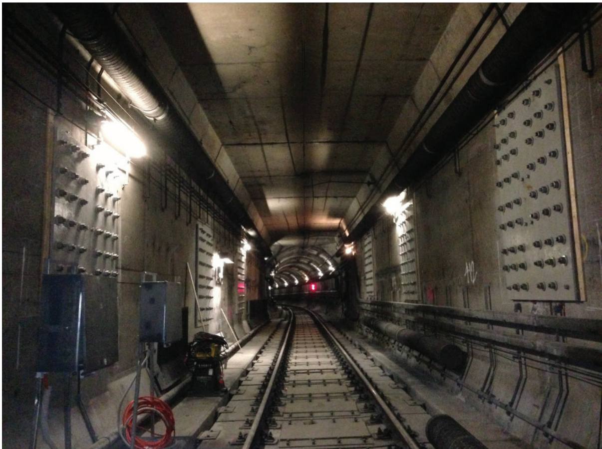
Figure 5: MURL tunnel completed strengthening works.
