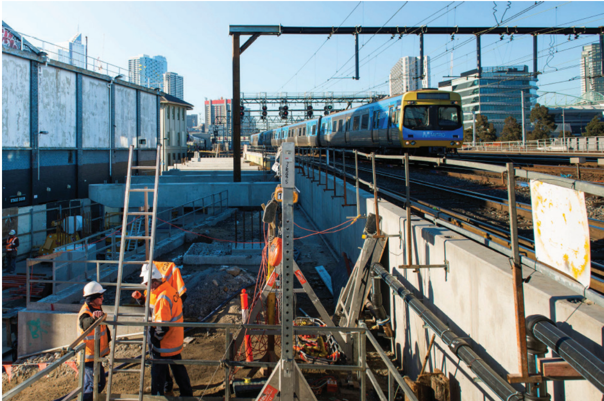
Figure 4: In situ column construction on Railway Place, directly behind Festival Hall.
