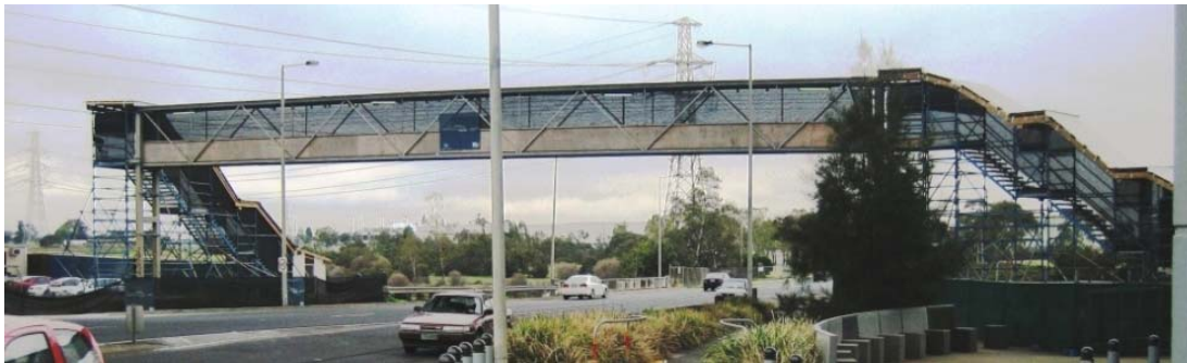
Fig. 8. Temporary Pier 10 (Hyde Street) Footbridge.
