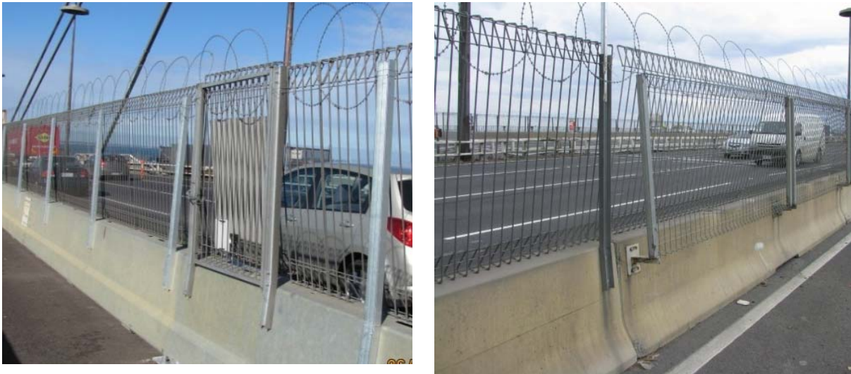
Fig. 6. Temporary steel (left) and concrete barriers (right) separating the construction lane
