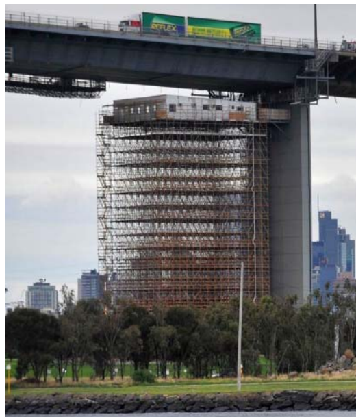
Fig. 9. Temporary Messing Facilities at Pier 15.
