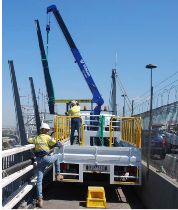
Fig. 12. Crane Truck in use in the Construction Lane
