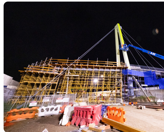
Above: Blaxland cable-stay bridge – temporary works
