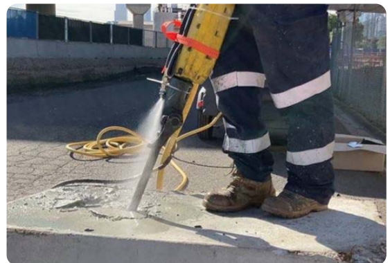
Above: A spray nozzle attachment suppressing jackhammer silica dust
