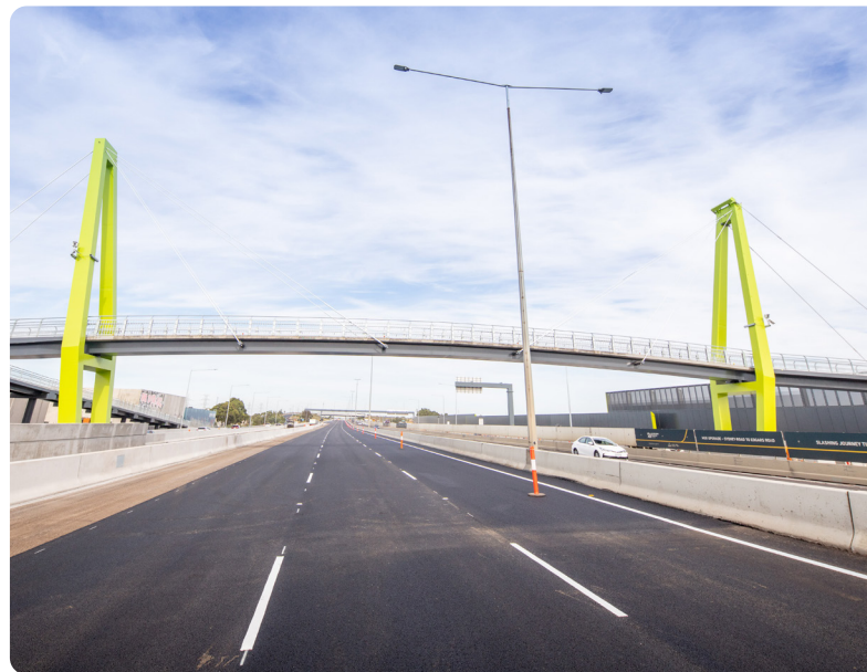
Below: Campaign style works allowed faster, safer and higher quality asphaltting
