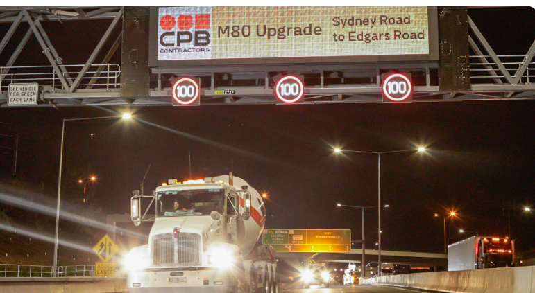
Above: Local steel fabricator Coslee supplied 70% of the project's gantries
