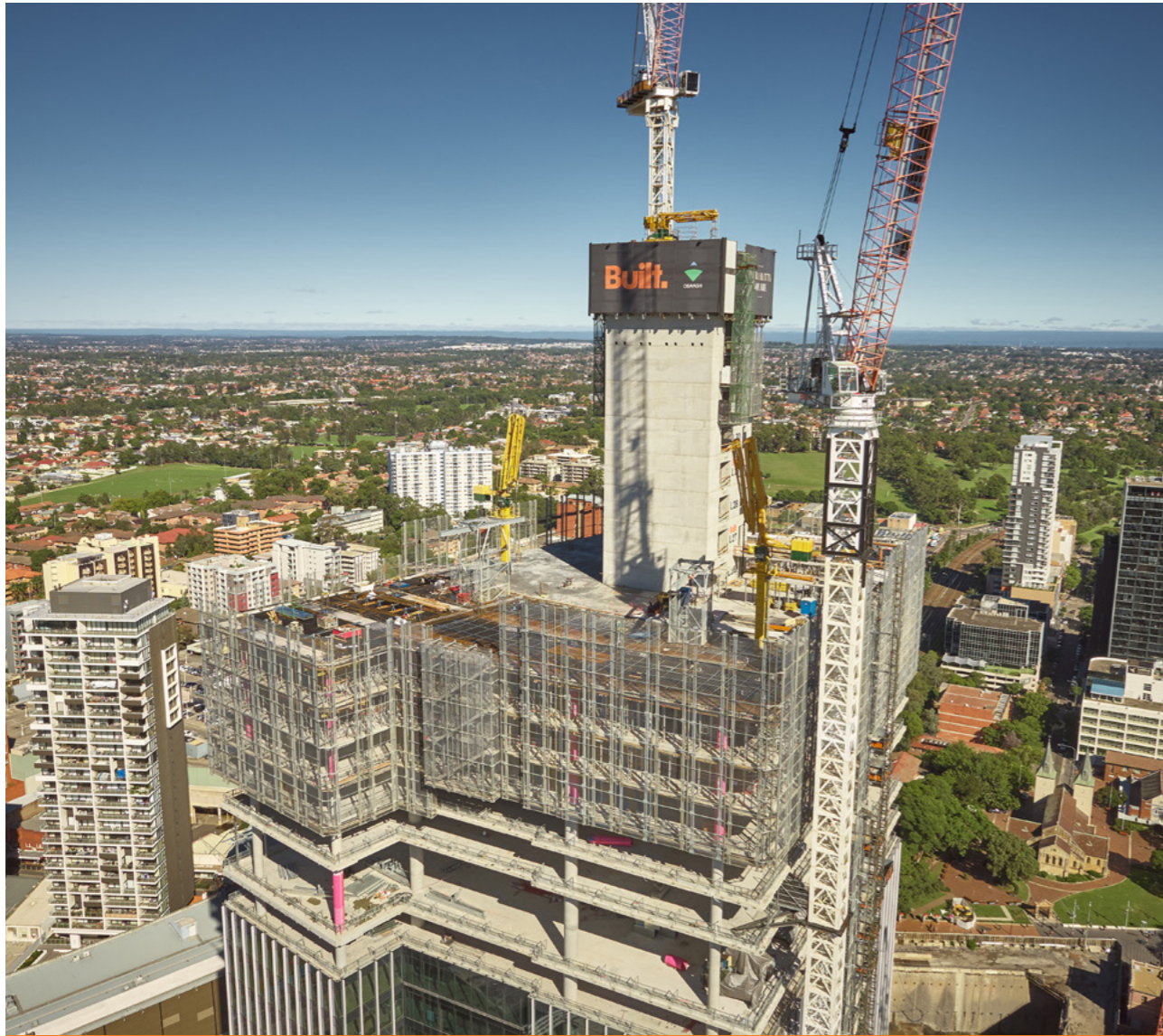
4PS jumpform system and form work hoists
