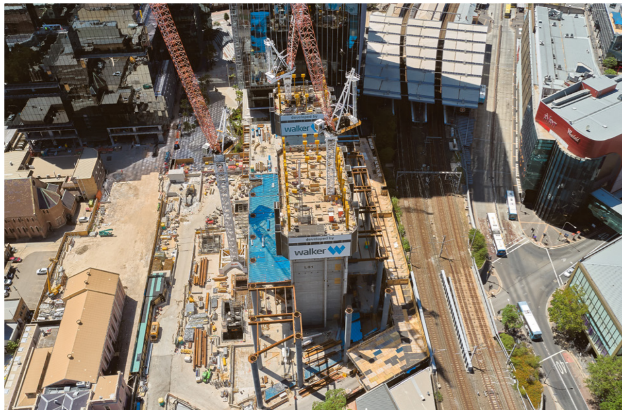
Reinforced concrete cores of towers 6&8
