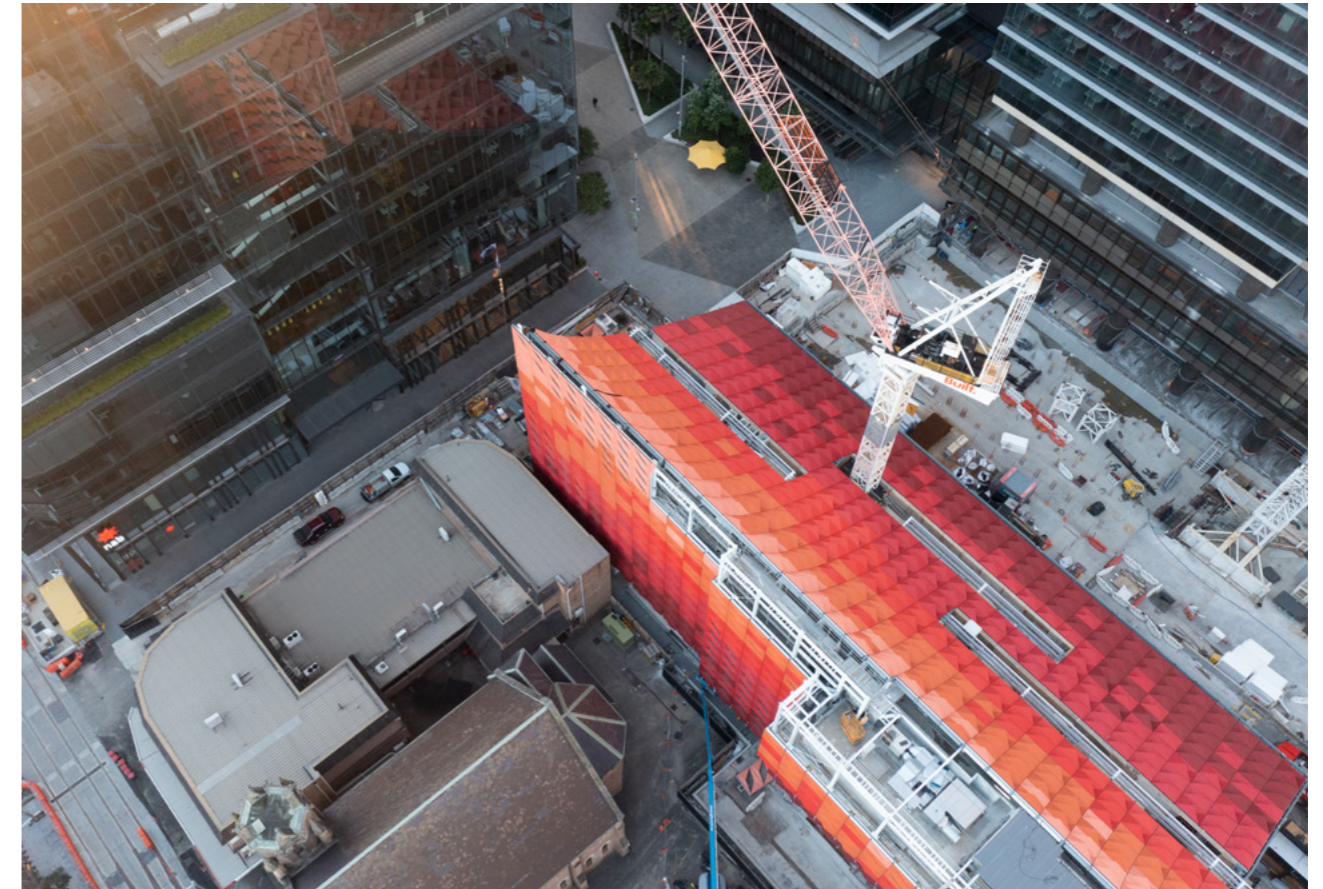
Cantilevered structure of PHIVE against the neighbouring buildings
