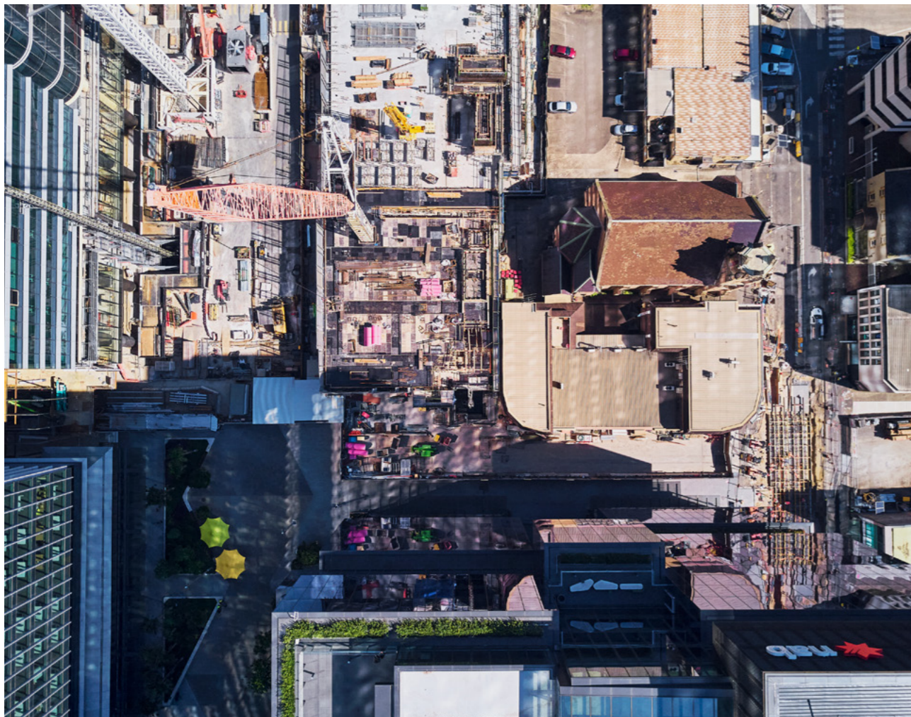
Tower crane and main core pad aerial view
