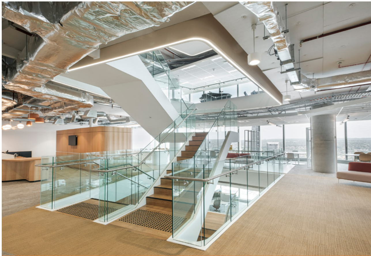
Above: 4PS final floor-to-floor height at 3.75m . Opposite: During and after construction of structural steel jump start methodology at 4PS
