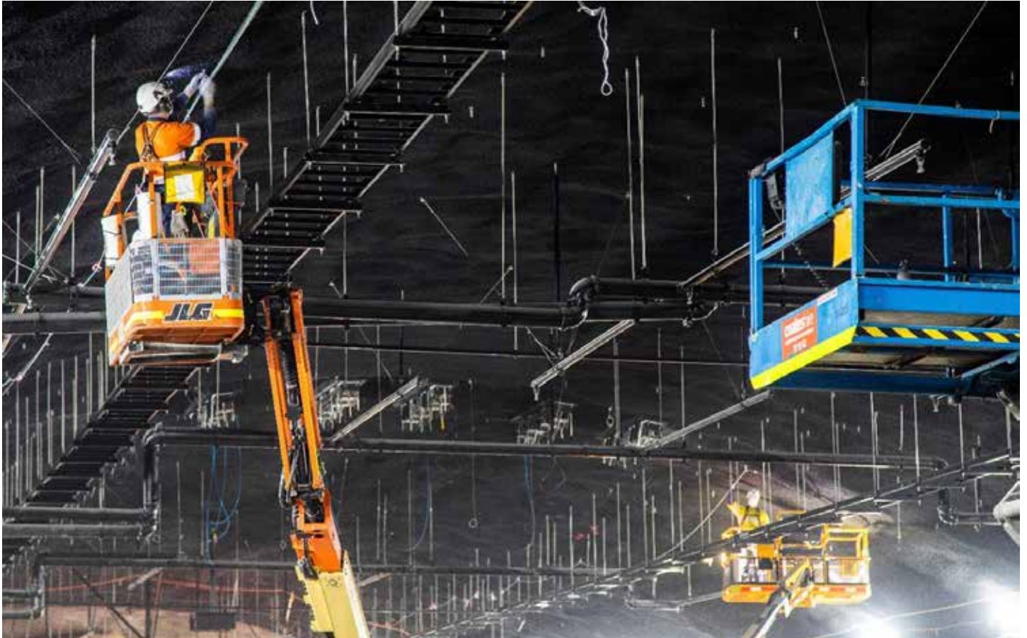
Installation of Mechanical and Electrical equipment
