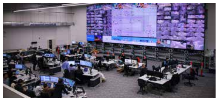
WestConnex Motorway Control Centre
