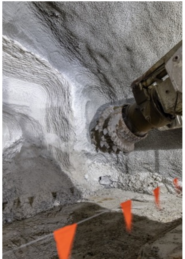
Roadheader breakthrough
