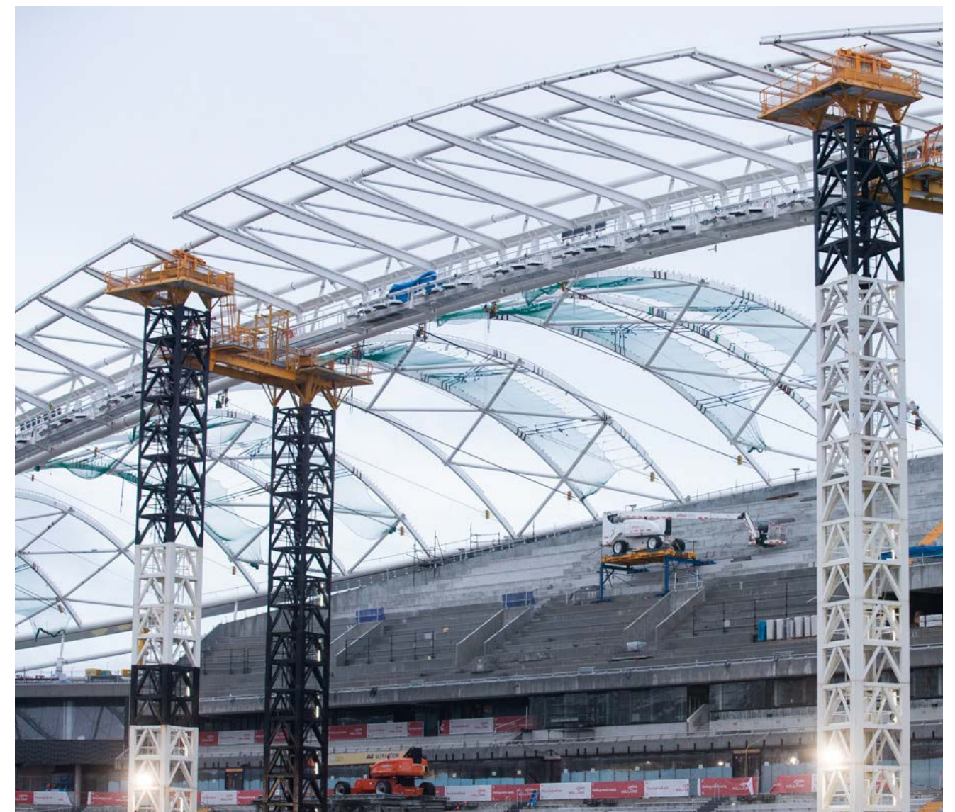
Temporary Headstock platform , with three truss sections positioned
