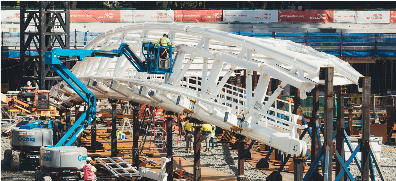
Truss sections being assembled on the pitch, dimensionally checked prior to lifting
